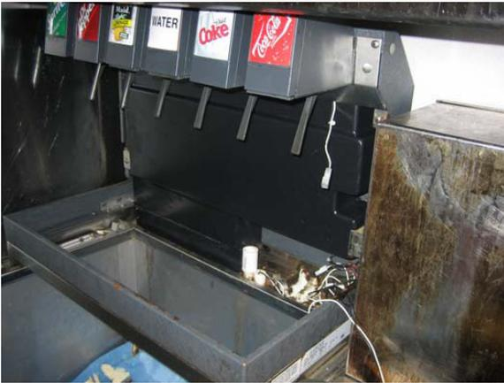
28. Install retaining brackets by first removing one of the screws holding the manifold tower to the tower cladding.
