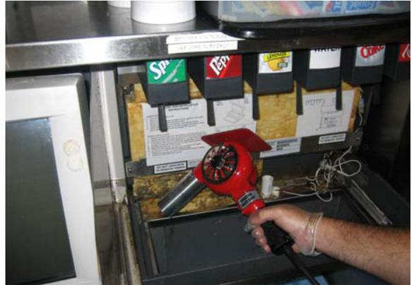
13. Trim the insulation according to images below (This shows the Lancer 6 valve Sabre which is the most complex to fit.)
