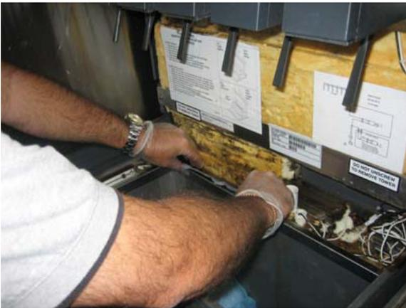
24. Rotate barrier into position, if necessary bending the left side out to slip it into place.
